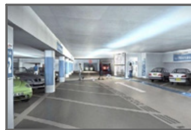
Parking souterrain de 1'100 places
